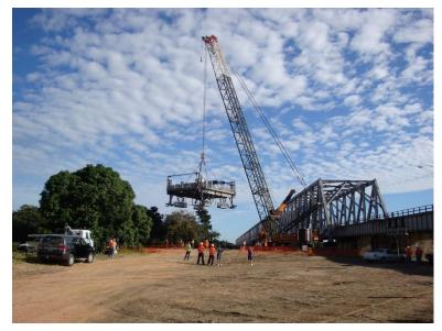
Structural repair works on the top structure of all ten spans and bottom structure of four spans are now completed.
